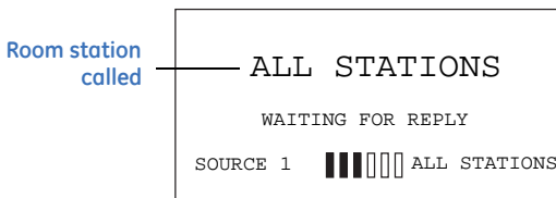
Figure 5. Calling room station Intercom screen
